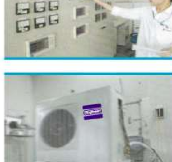
Noise testing Room (Indoor)
